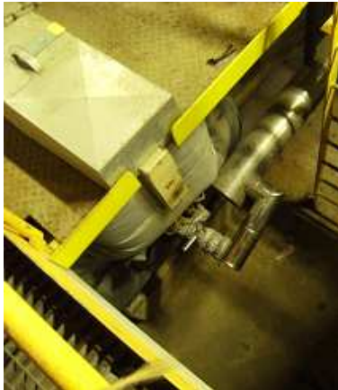
Fig 35a. Corner Taps on CoP 36" orifice meter. Fig 35b. Re-injection port downstream of plate.
