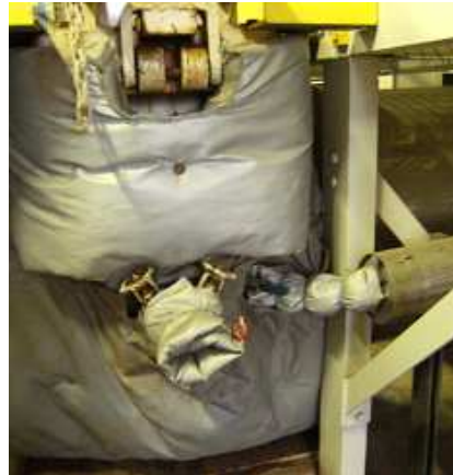
Fig 35a. Corner Taps on CoP 36" orifice meter. Fig 35b. Re-injection port downstream of plate.
