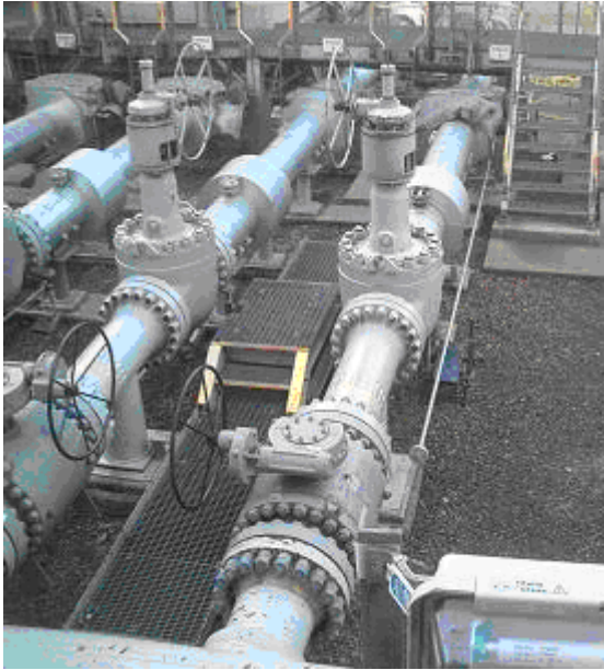
Fig 19. BP CATS upstream orifice run.
