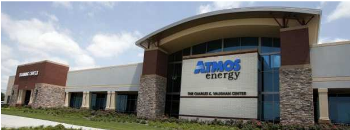
Fig. 1 The ATMOS Energy Corp. Training Center in Plano, Texas.
