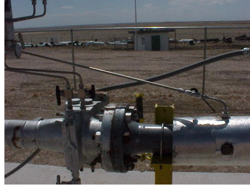
Fig 4. Orifice fitting with natural gas flow.
