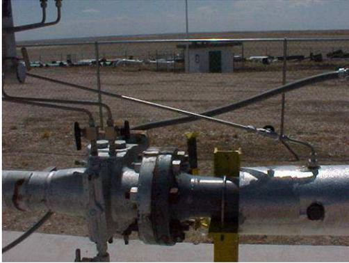
Fig 3. Orifice fitting with natural gas flow.
