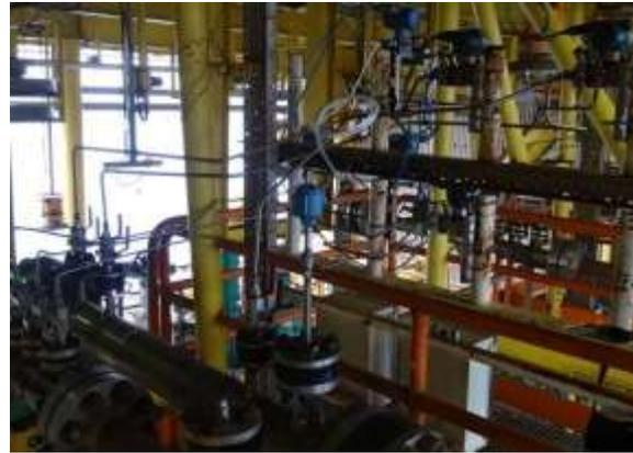
Fig 34. Venturi Meter Off-Shore in Malaysia.
