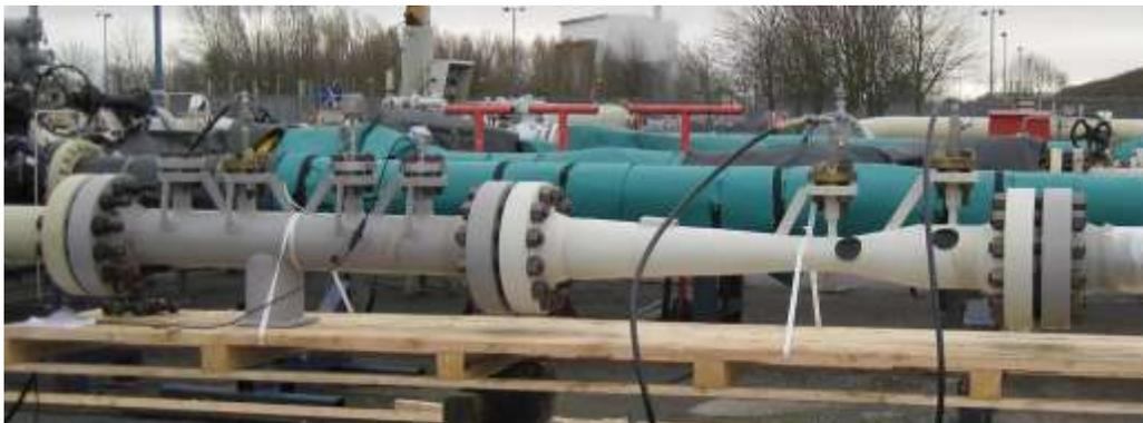
Fig 12. 8", 0.4 Beta Ratio Venturi meter (S/N 2009080-3) at GL Flow Centre
